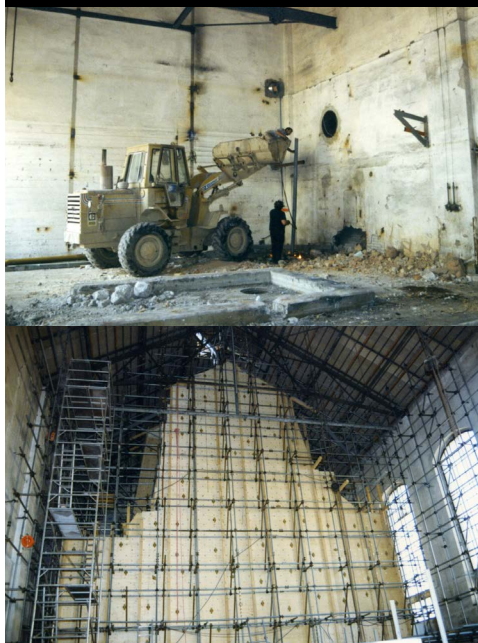
Halle 2: construction phases and Francois Legrand in 1996
